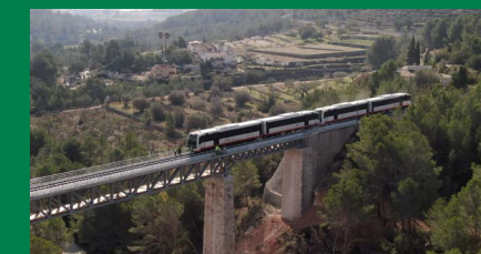
Rehabilitation Ferrandet Bridge Area I, East Management.
